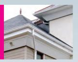
Any drainage system should have sufficient capacity to carry the expected flows of water at any point in the system. The actual flow in the system depends upon the area to be drained, the rainfall intensity and the position of the outlets.
